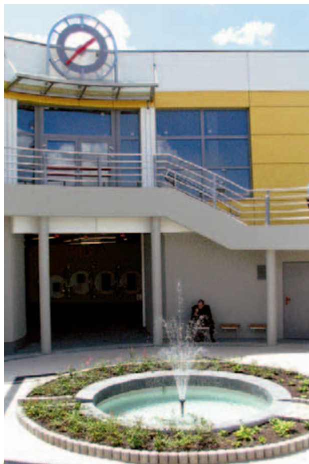
Atrium stanice Kobylisy.
